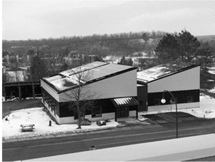
Figure 2: Finished Trent Forensic Crime Scene Facility. Source: Trent University. 2020.
