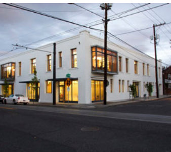
Lovejoy Office Building | Portland, OR Credit: Opsis Architecture
