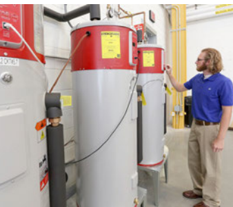
Maximum Energy Efficiency Research Laboratory Credit: Oak Ridge National Laboratory
