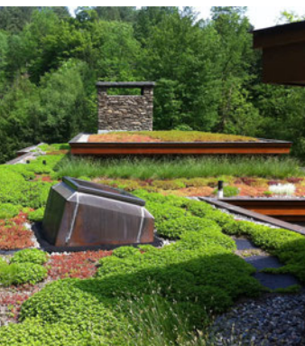
Maclay River House green roof | Moretown, VT Credit: Maclay Architects
