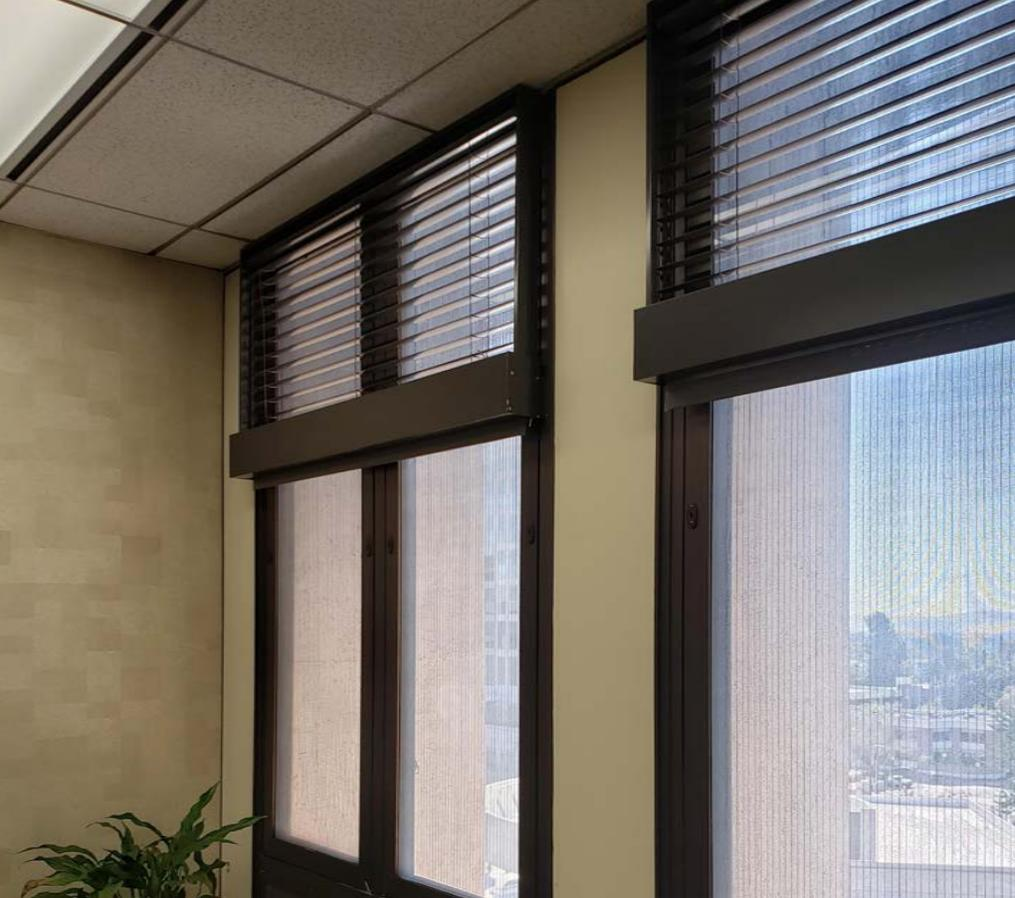
Upper blinds or lightshelves are independent of the lower shades and provide daylight that reduces energy use. Automated lower shades can be adjusted through the day, or during a meeting, to respond to occupant needs.
