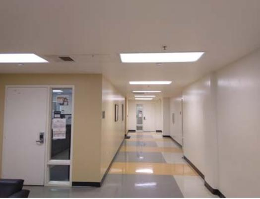
An office hallway with updated LED fixtures, occupancy sensors, wireless communications software and hardware, and improved monitoring capabilities. Credit: NBI
