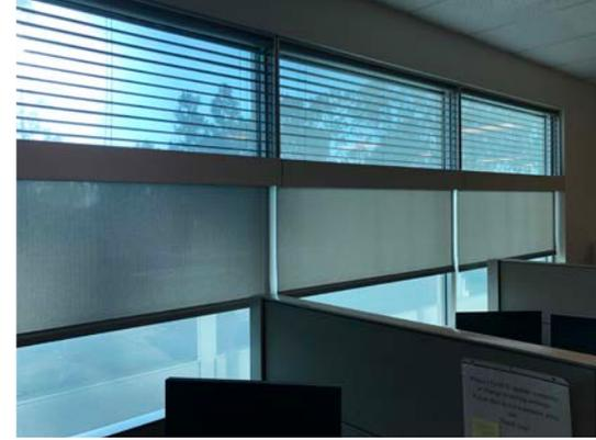
Upper blinds direct daylight deeper into the space. The lower shades provide privacy and daylight control. Credit: Rollease Acmeda Inc.
