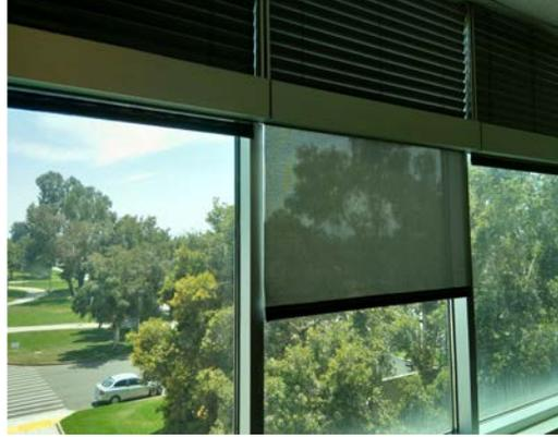
Upper blinds limit daylight while lower shades provide privacy while still allowing a connection to the exterior. Credit: Rollease Acmeda Inc.
