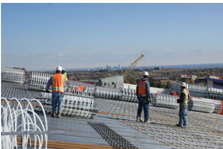
Custom-designed, rollout radiant tubing installation on site. Photo: Uponor
