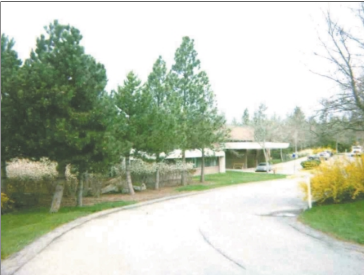
Spokane's Westlake State Hospital Retrofit
