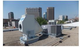
Evaporative indirect cooler that is integrated as a sidecar with an existing 5-ton RTU
